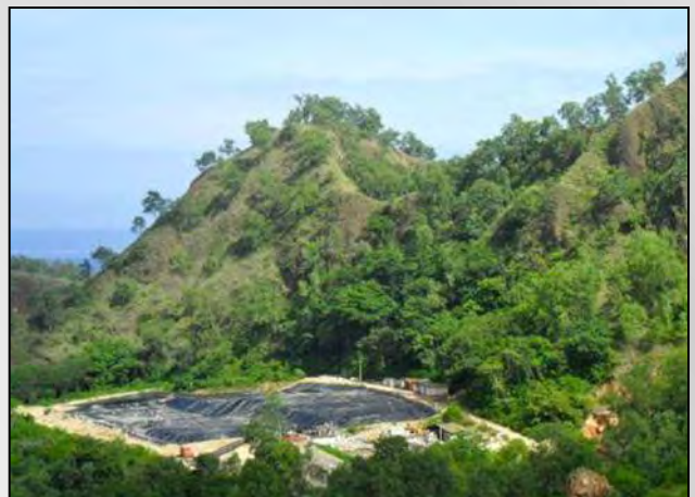
Fig 2: Demo Heap Leach with raincoats
