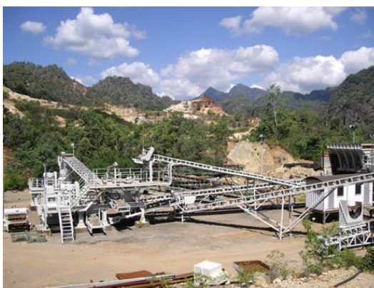
Fig 3: Refurbished crusher at Wetar
