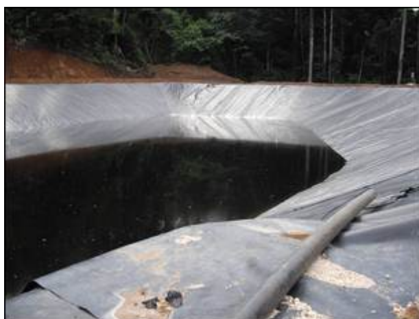
Fig 1: Completed new stormwater pond
