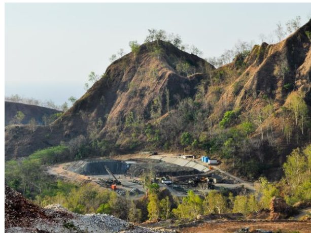
Fig 2. View of Demo Heap and Crushing Area
