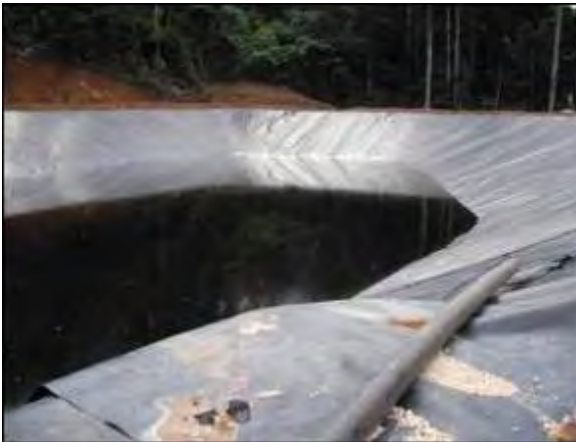
Figure 7. Completed new stormwater pond
