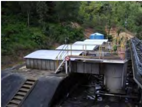
Figure 8. Covers on the SX plant
