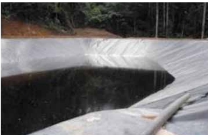
Figure 7. Completed new stormwater pond
