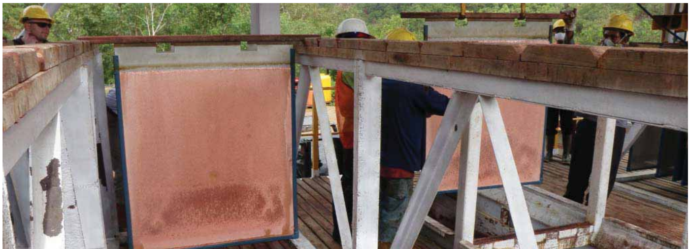
Stripping Copper Cathode at Demonstration Plant
